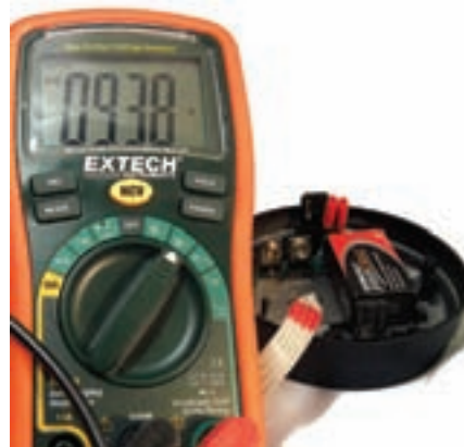
Figure 11. Voltage measurement with a diode bypass.
